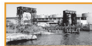
Decayed Gantry Post-industrial landscape, Bronx community's waterfront loss.
